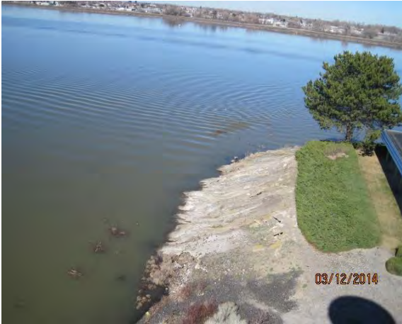
Area 1: Concrete spoils dumped at the northwest corner.
