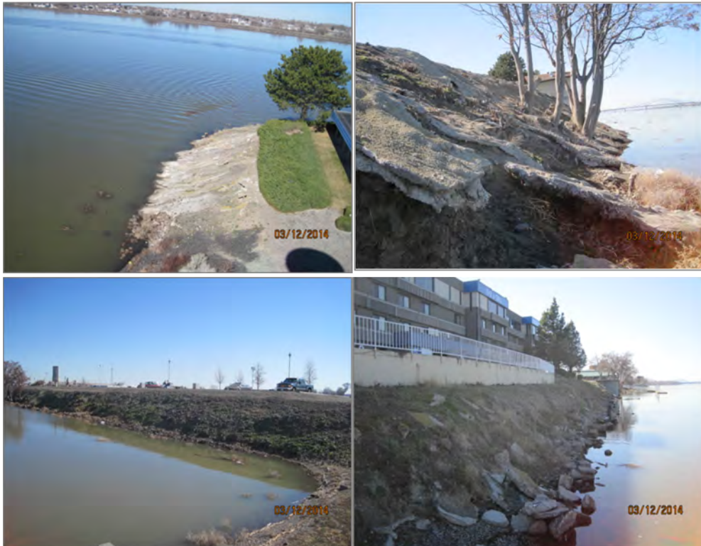
Figure 4. Examples of the present Clover Island shoreline exhibiting little to no riparian vegetation, steep, crumbling banks, and various concrete slabs and pours.
