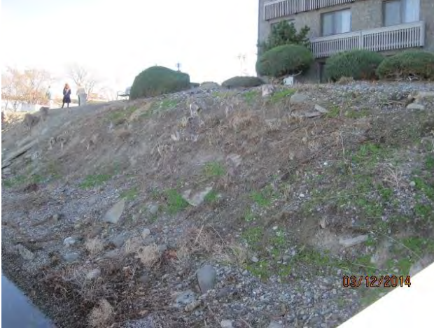
Area 4: Facing southeast
