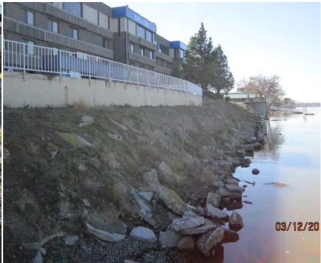
Area 4: Facing west.
