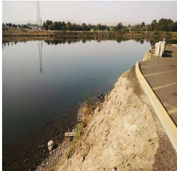
Figure 2-3 Erosion of Shoreline Abutting Parking Lot
